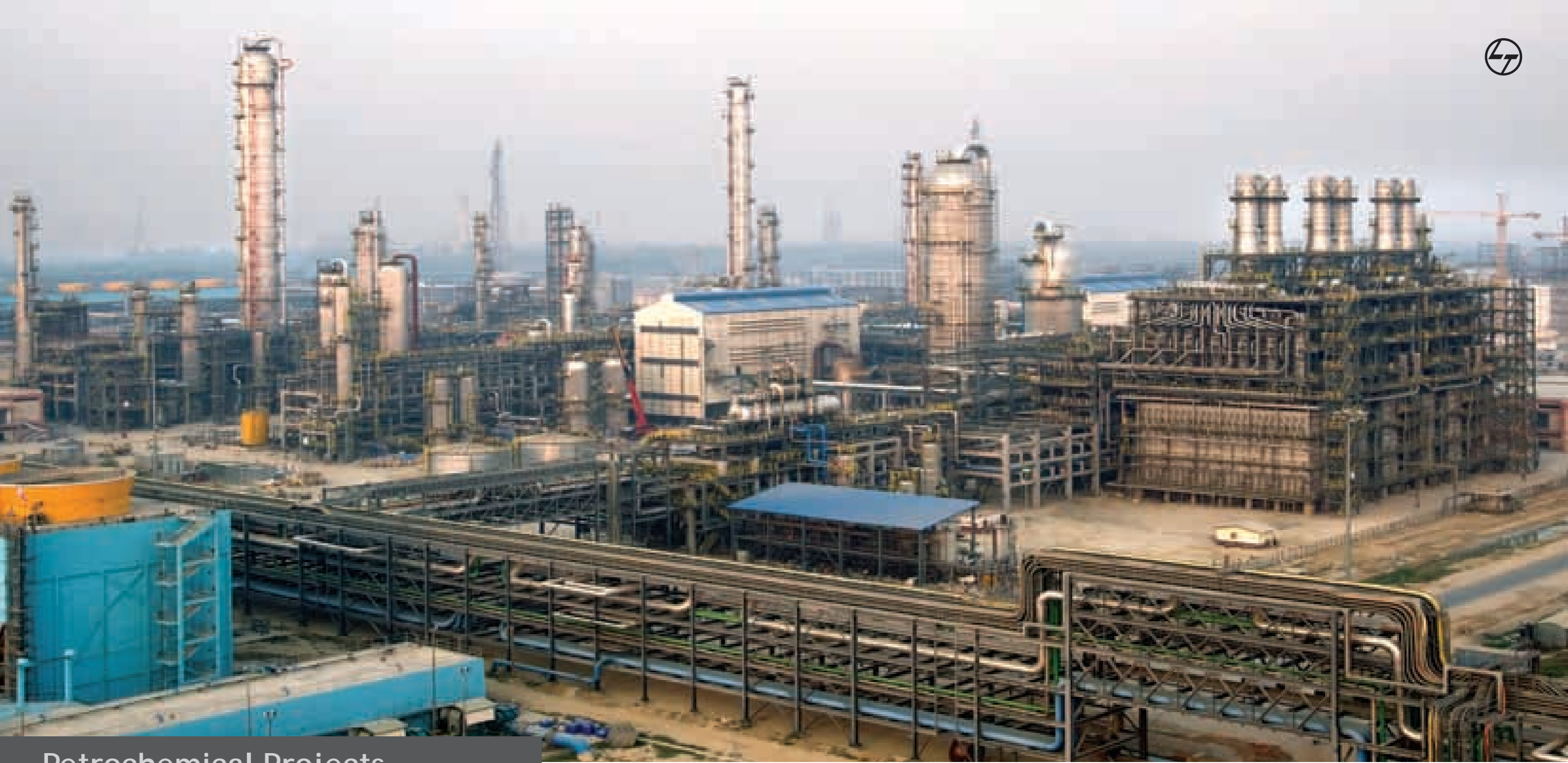
Cracking furnaces and associated units for IOCL at Panipat Naphtha Cracker Project. (Capacity : 800,000 TPA of polymer grade ethylene & 504,834 TPA of polymer grade propylene). L&T executed this project in consortium with Toyo Engineering, Japan.
