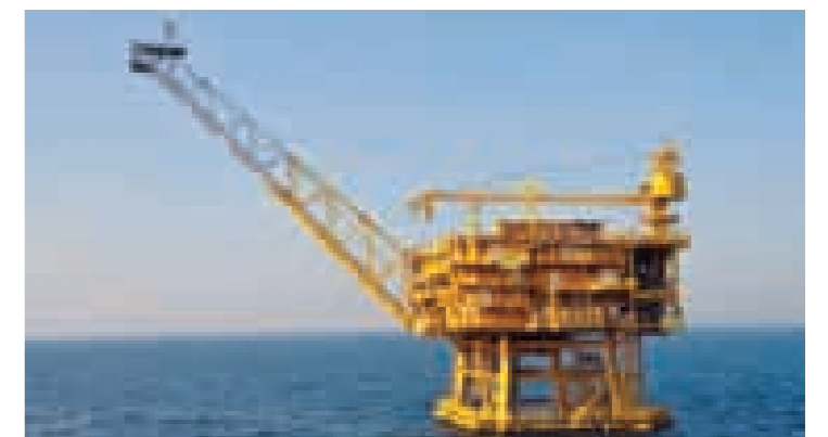
HA deck & building module for Maersk Oil - Qatar installed at Al Shaheen Field, off Qatar.
