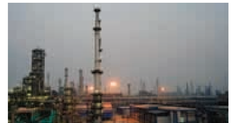
Motor Spirit Quality Upgradation Project executed by L&T for IOCL at Panipat. L&T also executed an MSQ project for IOCL at their Mathura Refinery.
