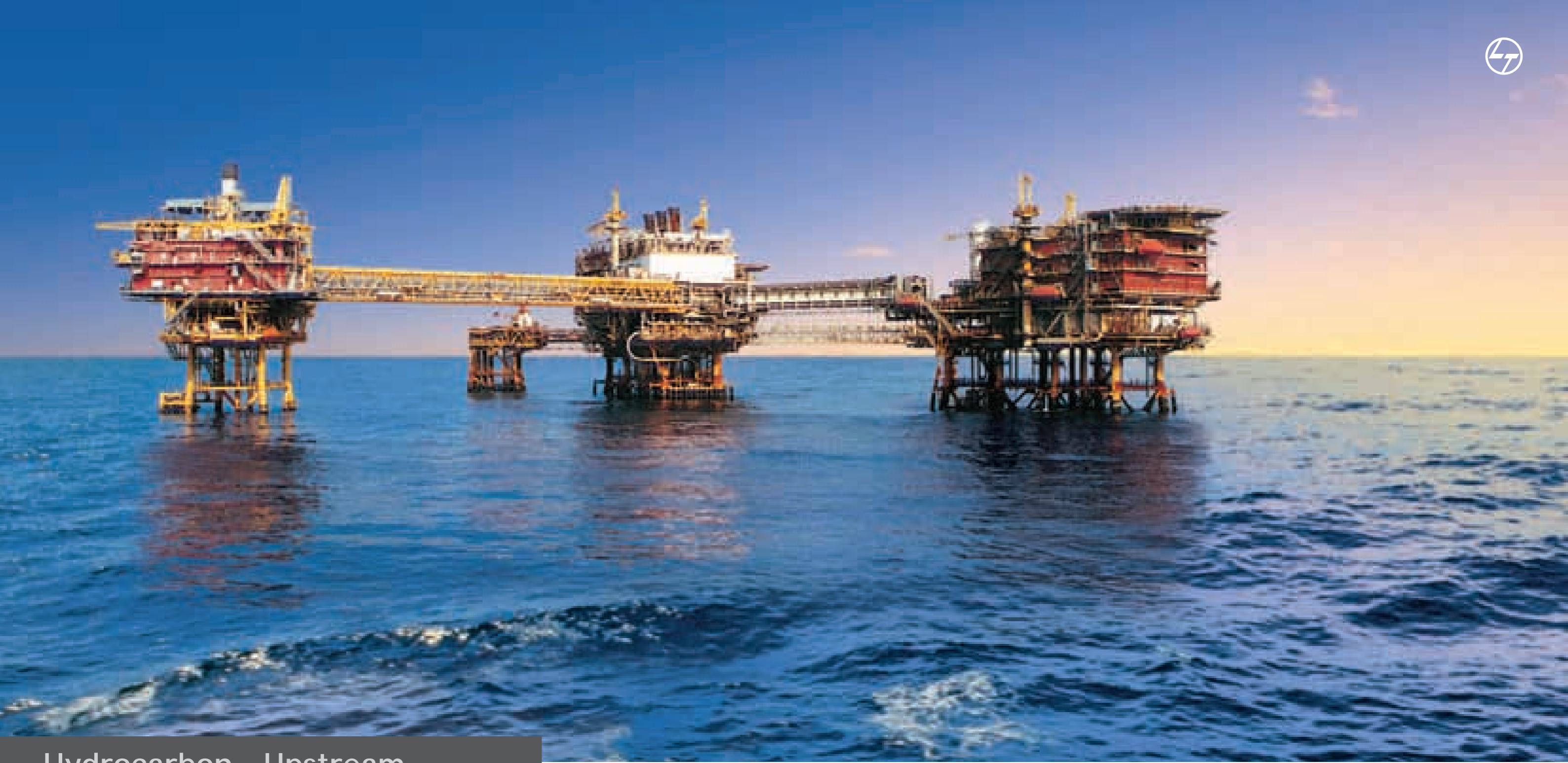
Process platform installation and pipeline modification at Heera Complex of ONGC (Capacity: 30,000 BPD oil, 20,000 BPD water, and 1.5 MMSCMD gas).
