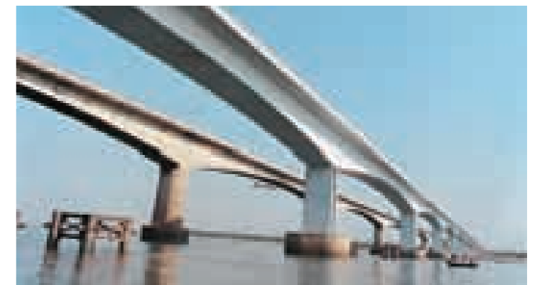
Bridge over the Narmada - built by L&T on a Build-Own-Operate basis.
