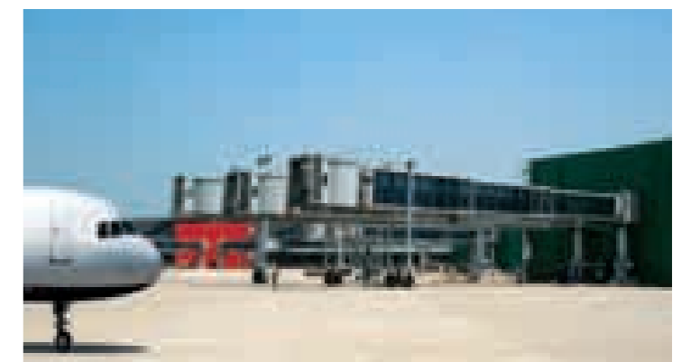
L&T's offerings in the airports segment include civil, mechanical, electrical and instrumentation, including all associated structures and airport systems meeting passenger amenities.
