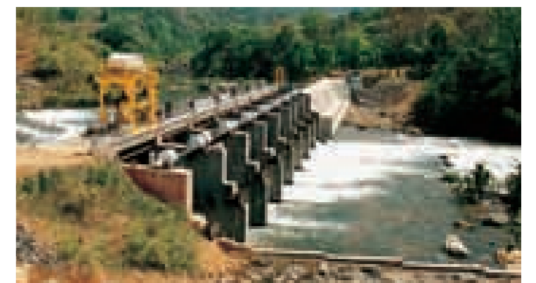
L&T offers comprehensive construction services for building hydropower projects.
