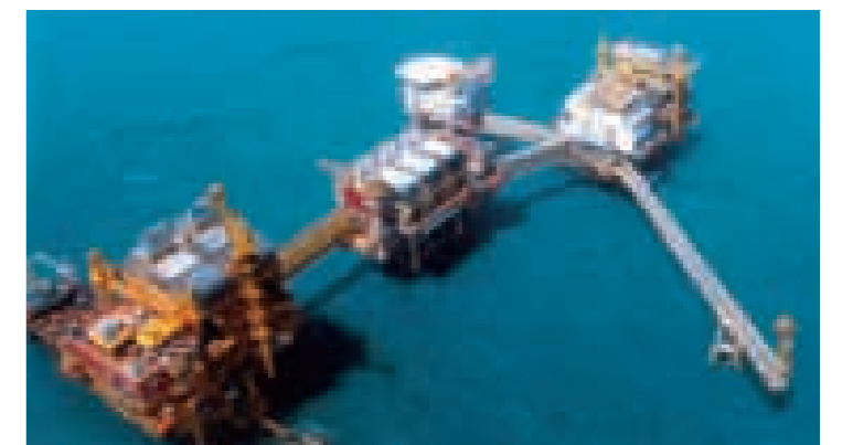
BCP-B2 Process Platform and Well-head Complex connected to the pre-existing BPB Complex of ONGC. It is located in the Bassein Gas Field, around 80 km north-west of Mumbai.
