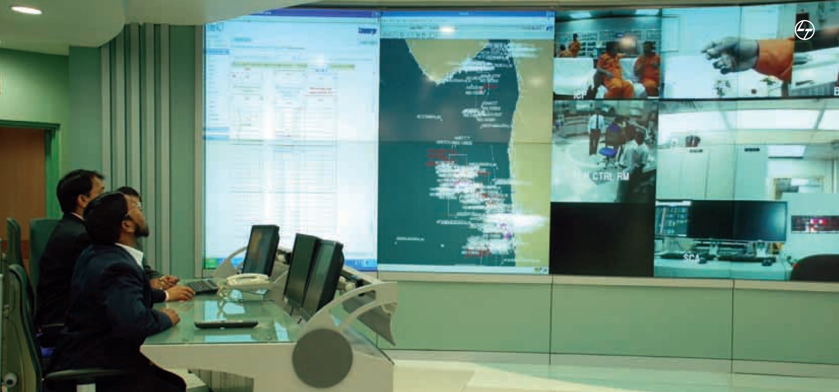
Supervisory Control And Data Acquisition system designed, supplied and commissioned by L&T for Onshore Control Centers (OCCs) for offshore operations of Oil & Natural Gas Corporation. The system connects 133 wellhead platforms, 13 process complexes and nine drilling rigs to OCC.
