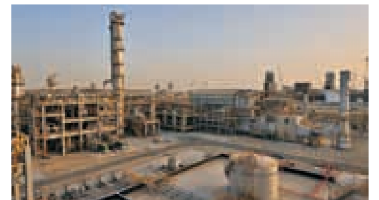
700 TPD Methanol & 100 TPD Carbon Monoxide Plant for Methanol Chemicals Company (Chemanol) at Al Jubail in Saudi Arabia.
